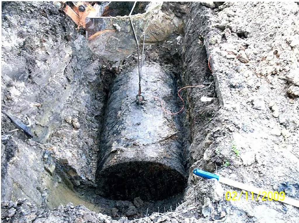
Picture 2: 113 Birch St. UST during excavation.
