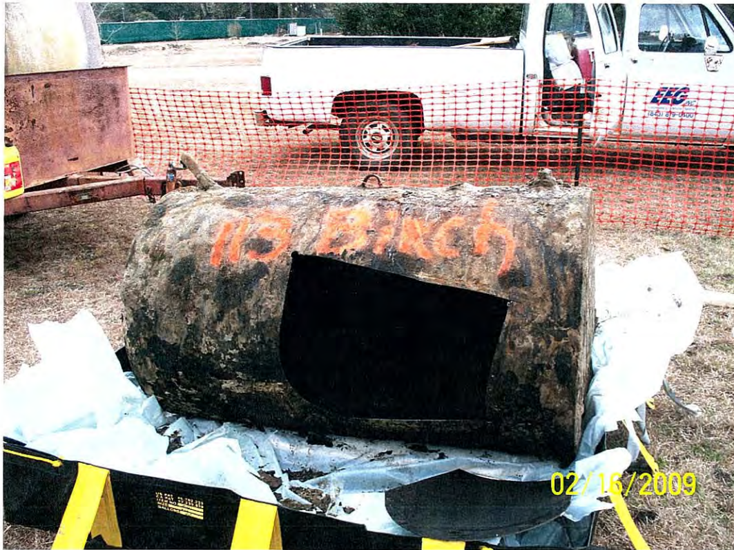
Picture 3: Demolition of tank in process.
